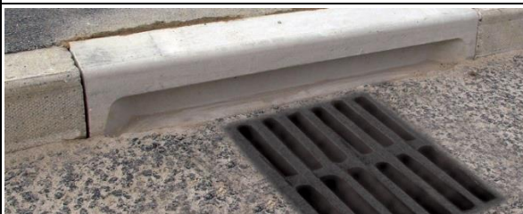
Example of a kerb designed to allow amphibians to bypass gully grating
